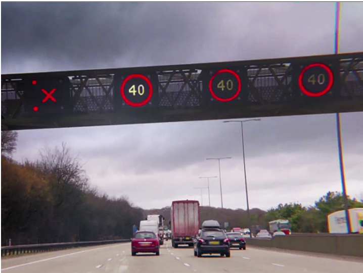
Figure 5 - Auto-enforcement of Red 'X' signs
